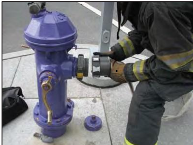
Hydrant Adaptor used to connect LDH to the hydrant.
