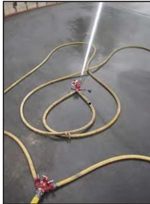
Charged Monitor Manifold.
