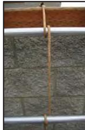
The rope is then brought behind the second rung below the sill/wall/roof line
