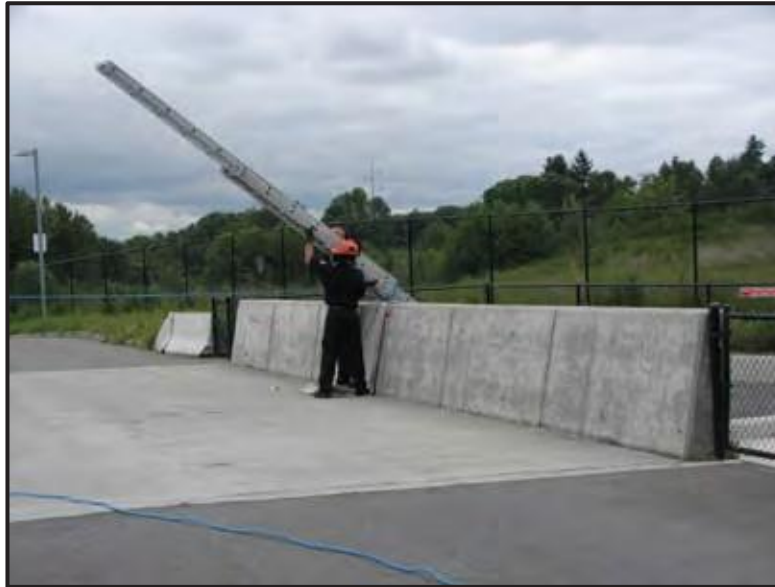
As the ladder reaches its fulcrum, assist the ladder from not slamming into the wall/building
