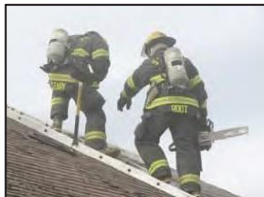
Members standing on and working from a roof ladder
