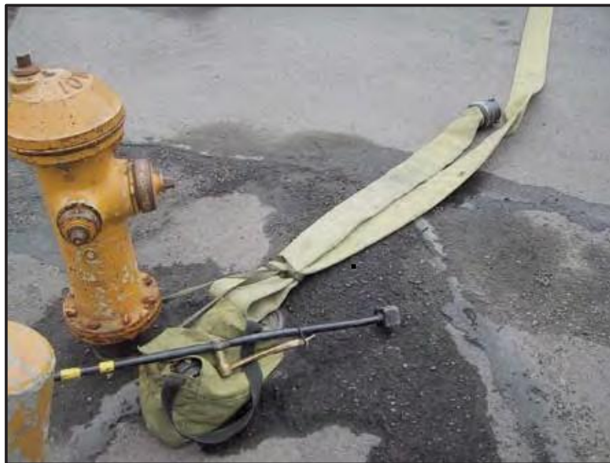
Hydrant tools and LDH waiting for the second engine to make the connection.
